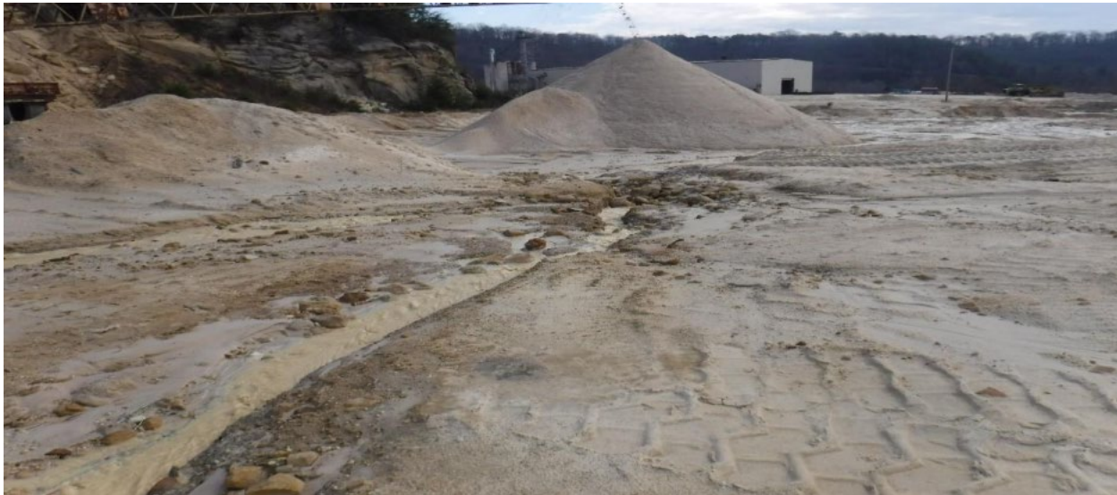
Photo 6 - Wash plant process wastewater discharge to stormwater outfall 004.
