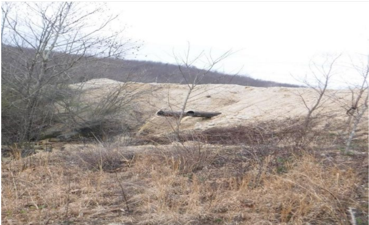
Photo 12 - Outlet/discharge pipes from upper pond.
