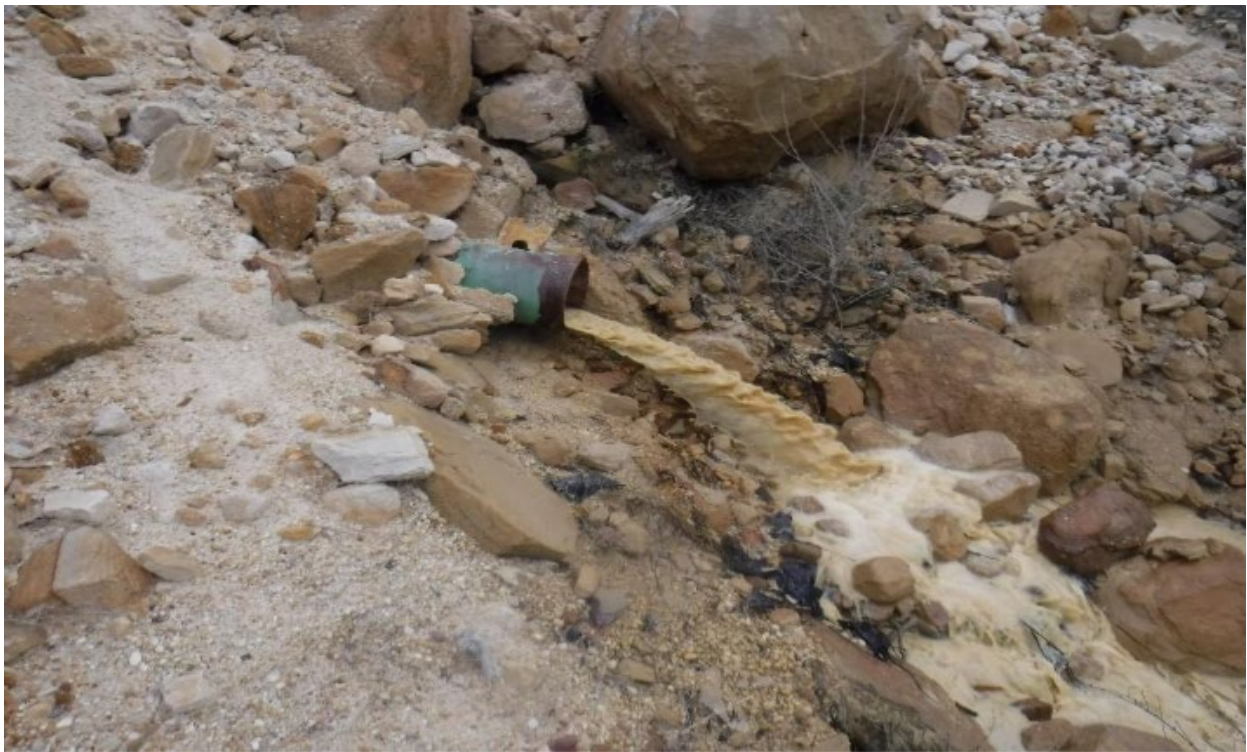
Photo 4 - Stormwater outfall 004 discharging process wastewater from wash plant.
