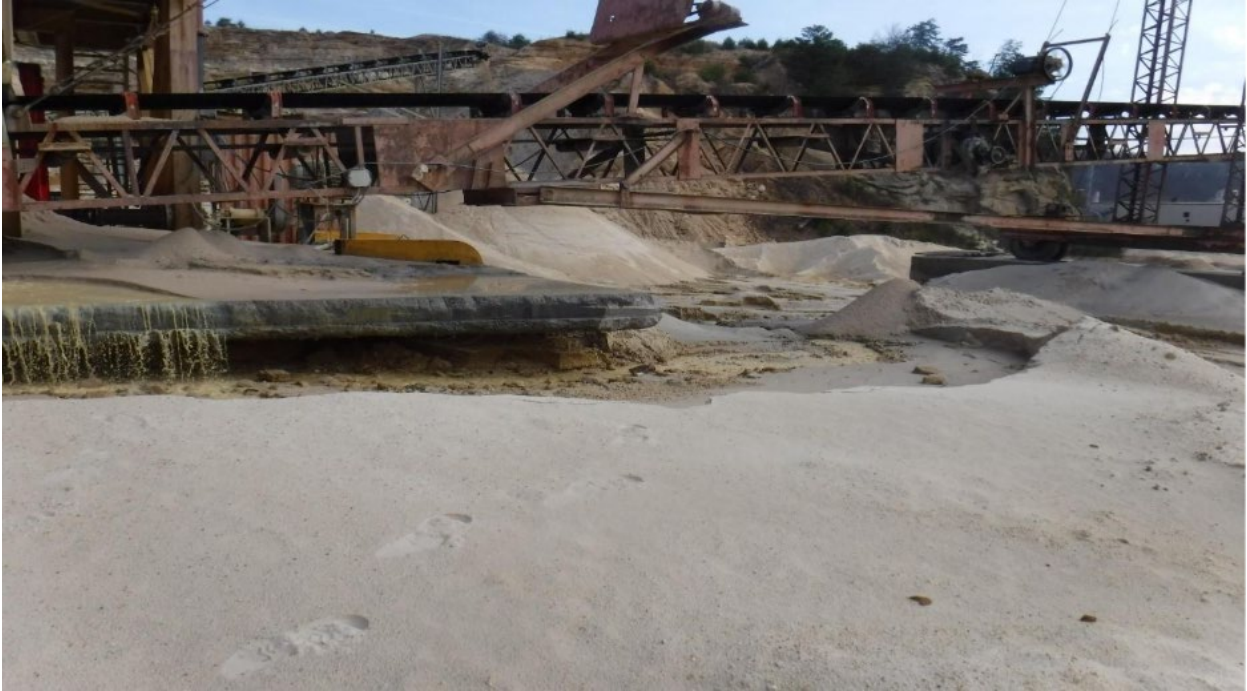
Photo 7 - Wash plant process wastewater discharge to stormwater outfall 004.
