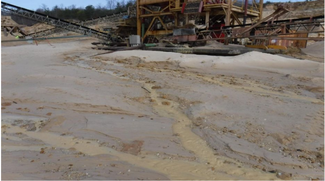
Photo 5 - Wash plant process wastewater discharge to stormwater outfall 004.
