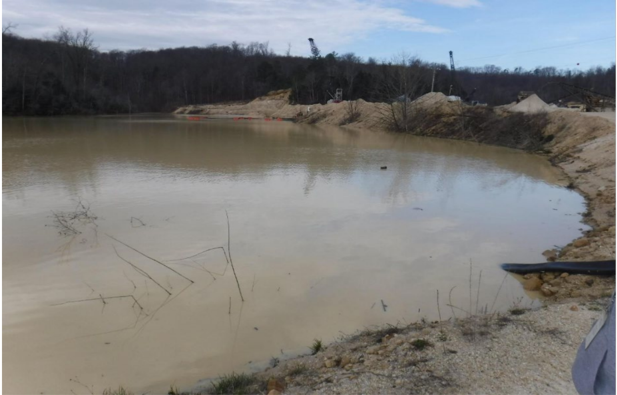
Photo 11 - Upper pond- side near outlet/discharge pipes for upper pond.
