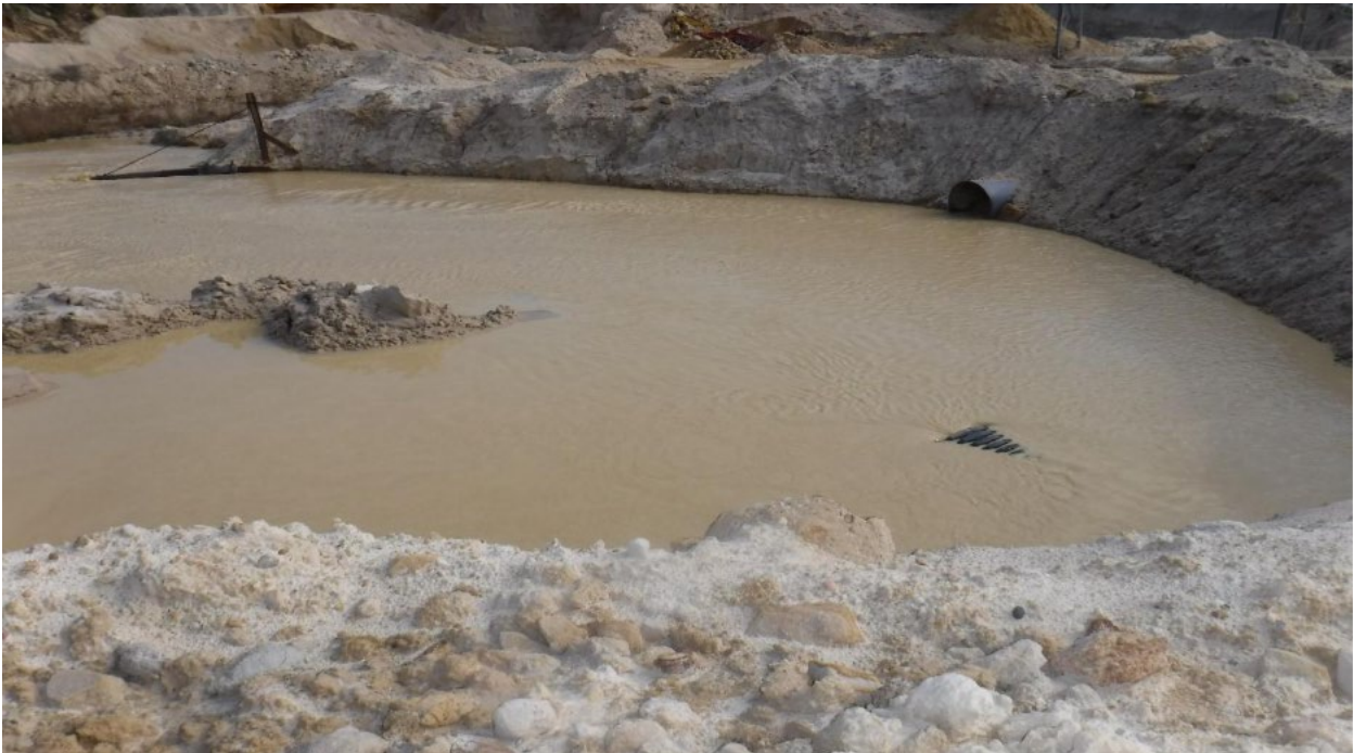
Photo 8 - Process wastewater treatment cell 1 inlet and outlet pipe.
