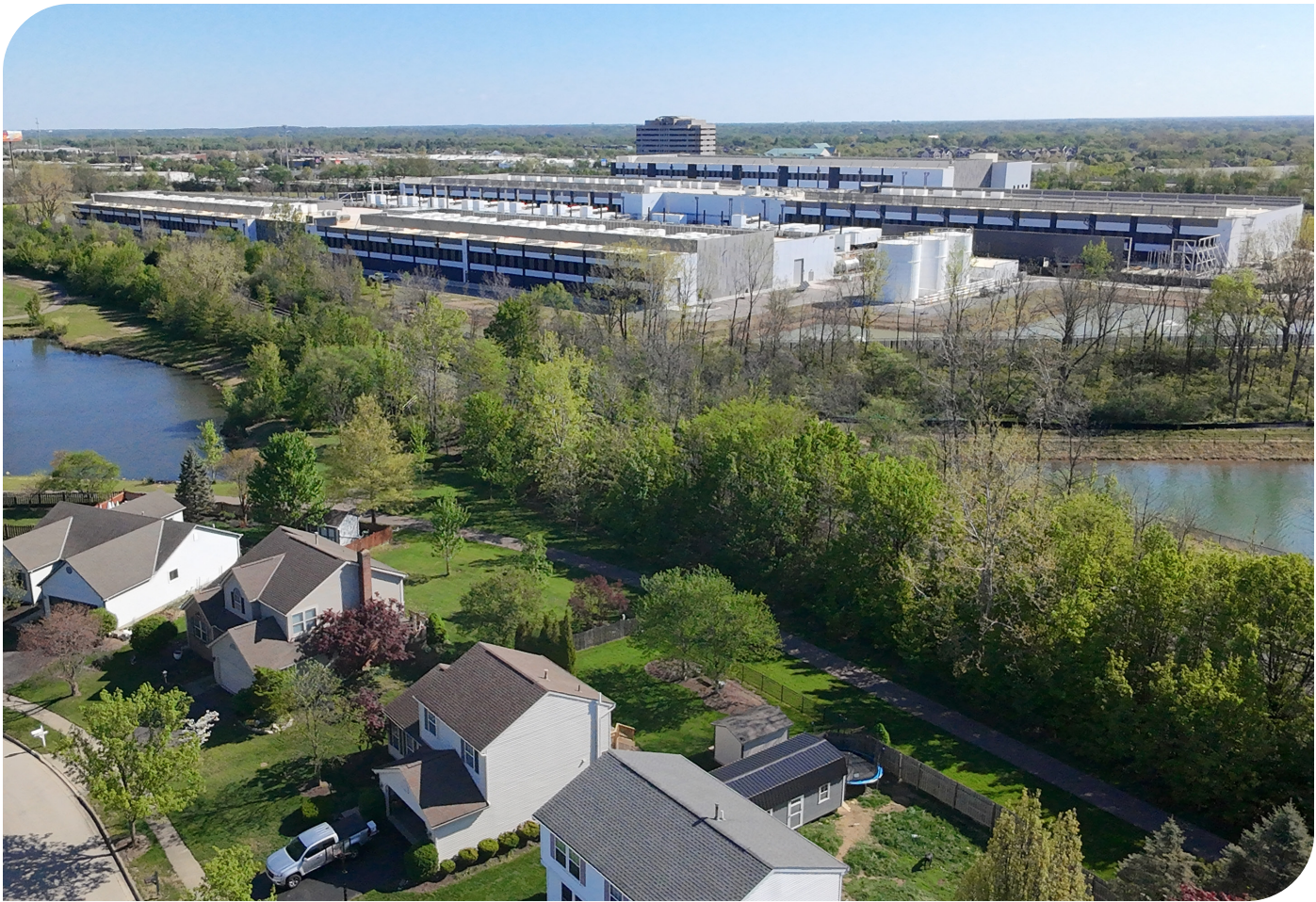
The Amazon data center on Scioto-Darby Creek Road sits directly next to homes in Darby Glen subdivision in Hilliard.
