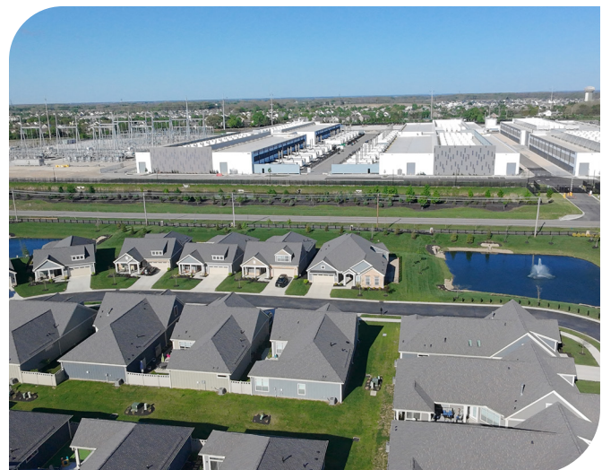
An Amazon data center sits directly across Leppert Road from homes in the Carr Farms neighborhood of Hilliard.
